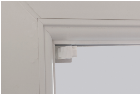
4. Check bracket is squarely secured. Repeat both sides.
