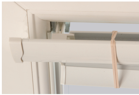
14. With rubber bands in place, align the headrail end cap slot with bracket arms.
