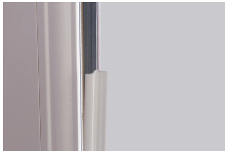
8. Place the side profile* against the side frame with flat face towards the glass and the notch to the bottom.
