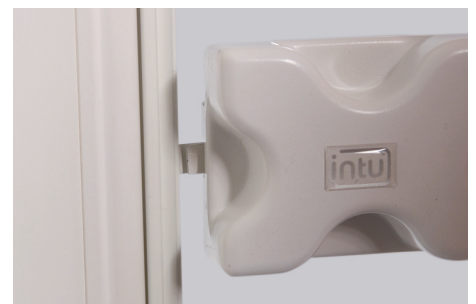
12. Press home using the insertion tool. Fully located the clip will sit over the side profile.
