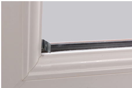
7. Check bracket is vertically secured. Repeat both sides.
