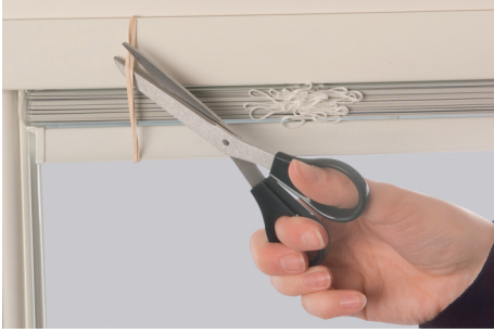
16. Snip off the rubber bands and carefully lower the slats to the bottom frame.
