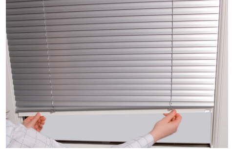
18. To align the bottomrail horizontally, simply pull it into the position desired. It will stay in position under tension from the cords. Align bottomrail to the horizontal.
