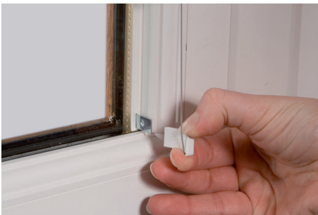
17. With cord at bottom of bracket, slide onto clip. Repeat both sides.
